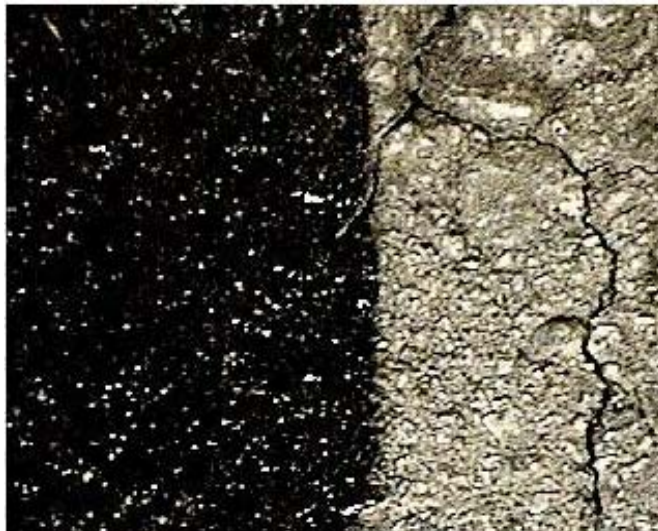
Figure 11. Effects of Oxidation on ACHM
